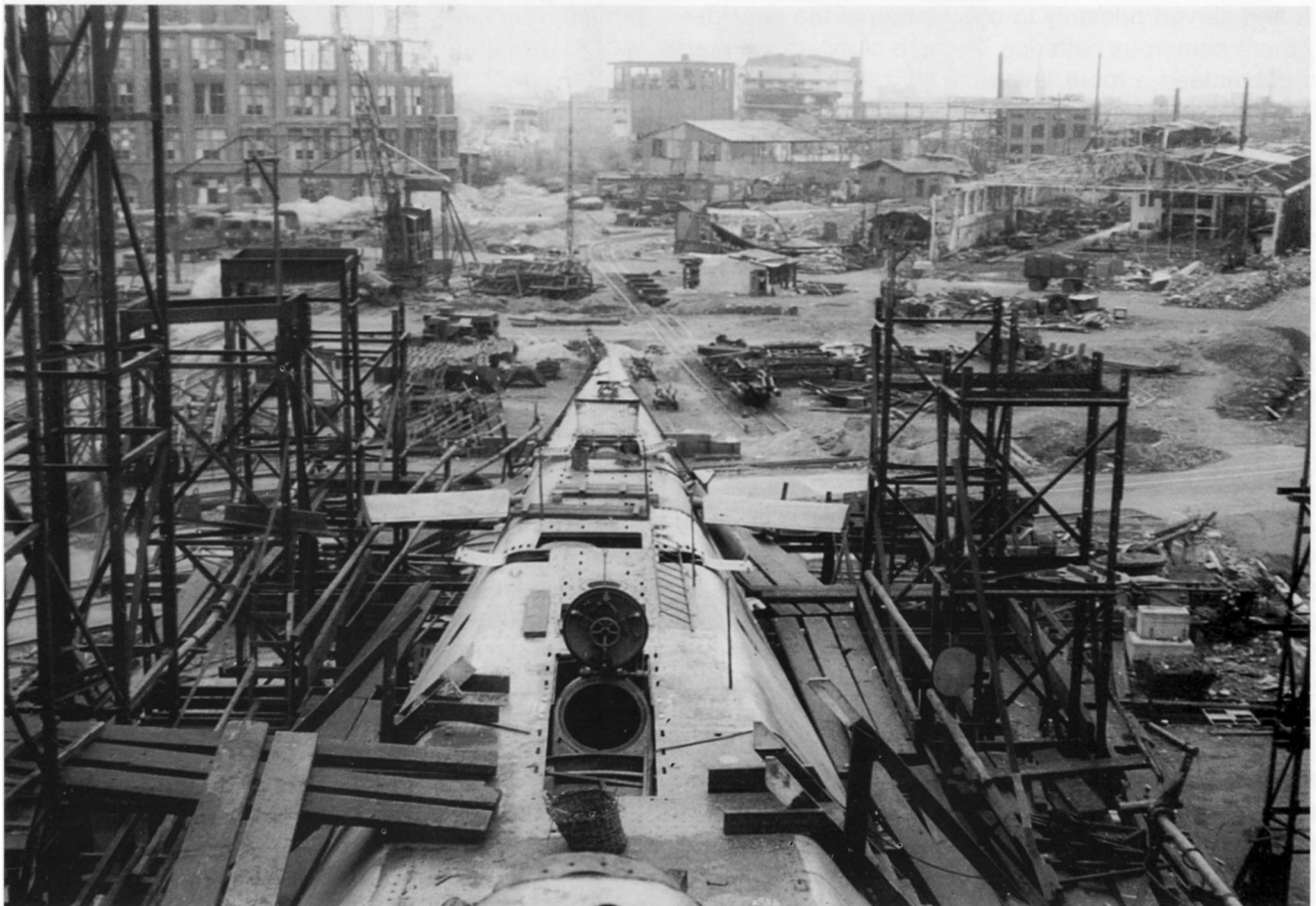
Below: The Blohm & Voss shipyards just after the war ended. Here the rear of a Type XXI U-boat is ready to be assembled.
