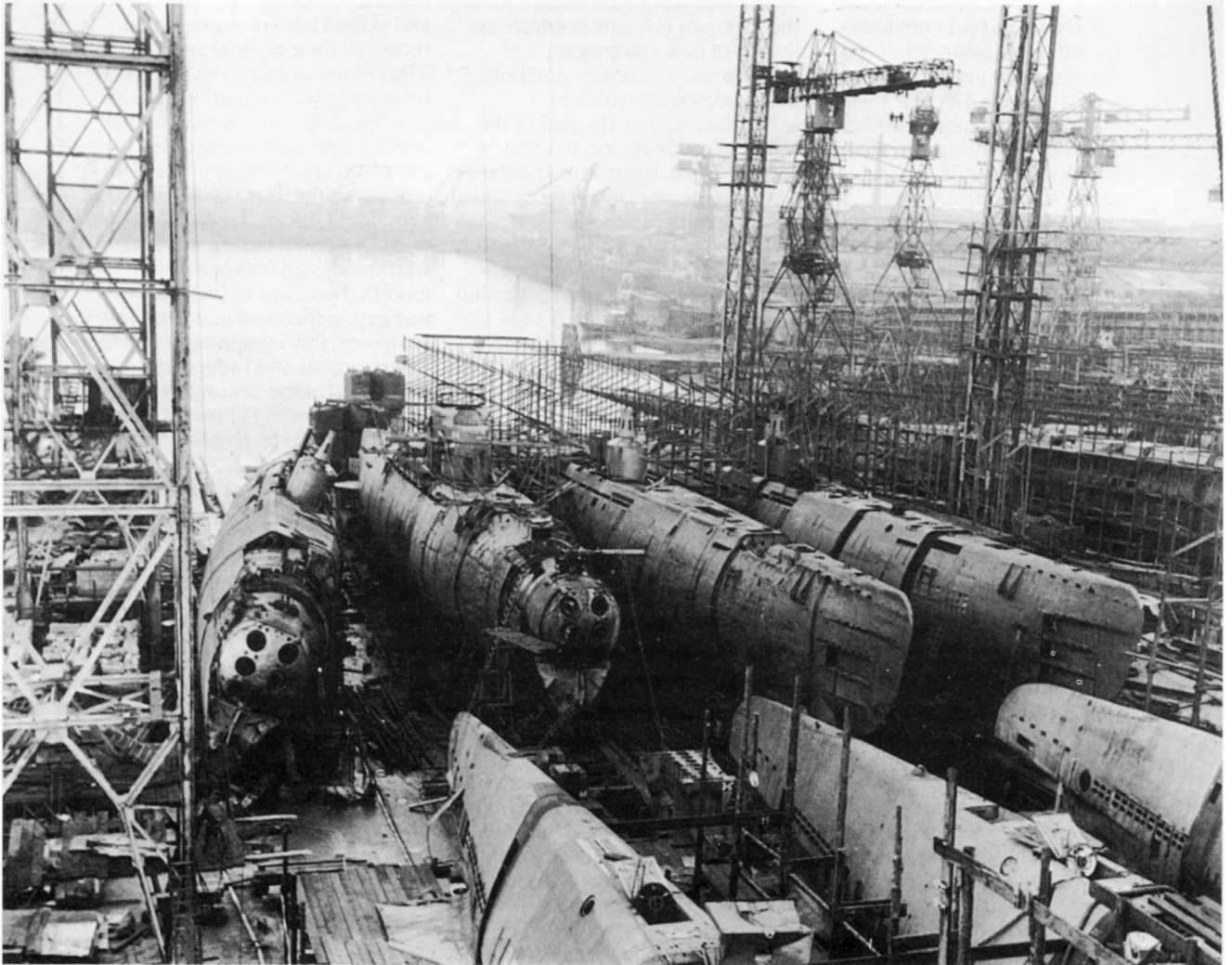
In this picture—taken a few days after the armistice—the series production system of the Type XXI U-boats is clearly shown. While several U-boats are ready to launch in front, the next ones are taking shape behind them, to be launched in turn. At left is a boat that fell victim to bombing, tipping on its side. The picture shows the Deschimag shipyard in Bremen, one of the three shipyards where this type of U-boat was built.
