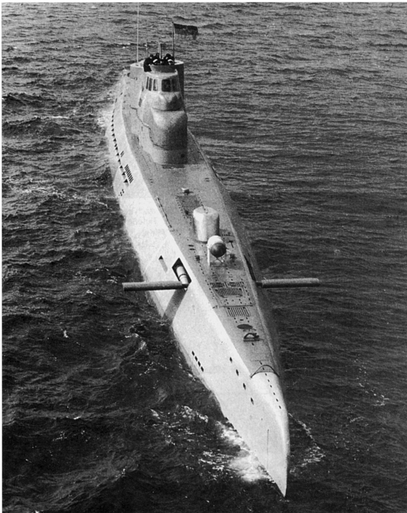
U 2540, sunk by its crew on orders at the end of the war and raised in 1957, was used by the postwar German Navy for many years as the test vessel after rebuilding, with its forward depth rudders extended.
